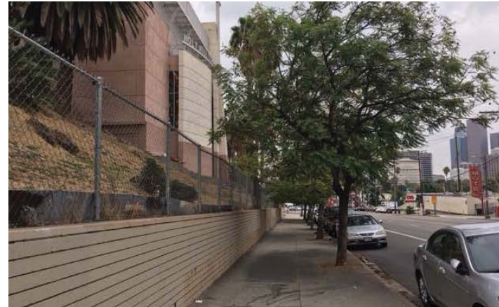
View of the eastern sidewalk of Sunset Boulevard adjacent to the property site, viewed southwardly from its intersection with White Knoll Dr.
